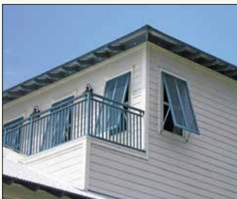
Figure 4-11. Bahama shutters made from durable extruded aluminum components add "islands" flair to a home and provide effective opening protection. Image courtesy of Roll-a-way.
