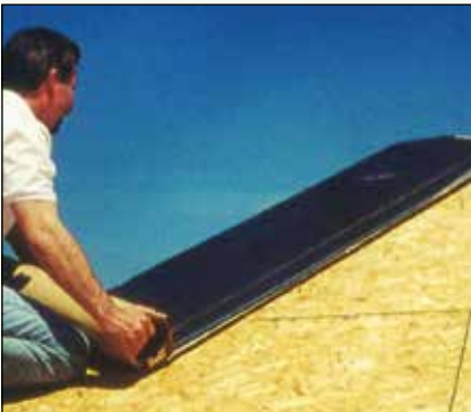
Figure 4-8. Synthetic underlayments are typically made from polypropylene, polyester, or fiberglass fabric, which weighs less than felt building paper, can be manufactured with anti-slip surfaces, and can withstand exposure to the elements for six months. Image courtesy of Carlisle Coatings & Waterproofing.
