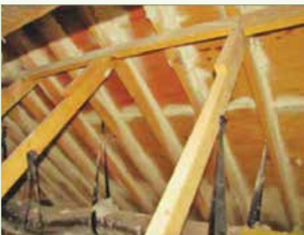
Figure 4-5. Spray polyurethane foam is used to add strength between the rafters and the plywood sheathing. This method can be used to strengthen existing roofs and may negate the need to replace older roofs. It can also be used where fasteners are missing or at the corners of hip style roofs or the ends of gable end roofs, which are especially susceptible to wind forces. See FEMA publication numbers P-499 and P-804. Image courtesy of FEMA.
