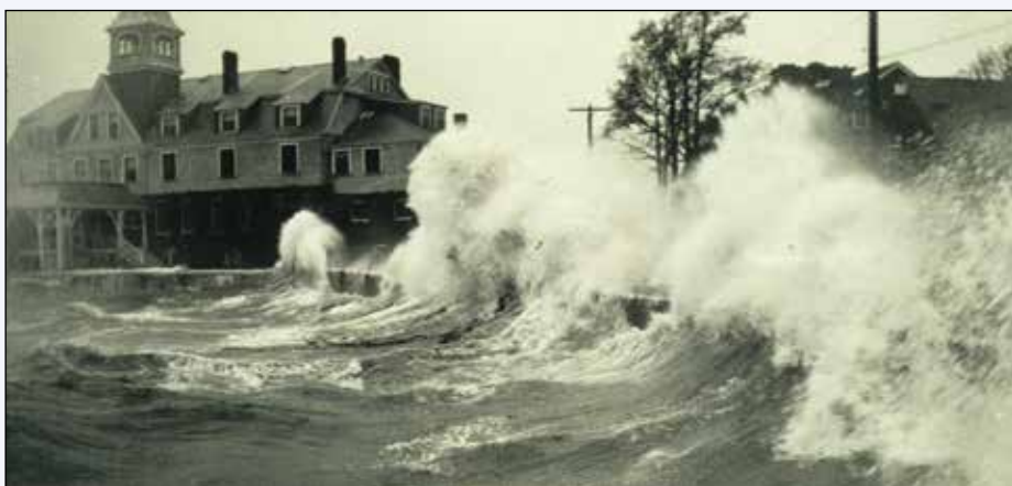
Figure 2-4. The south side of Main Street, Woods Hole, MA during the 1938 Hurricane. Bureau of Commercial Fisheries building on left. Photo Credit: NOAA Photo Library, NOAA Central Library; C&GS Season’s Report Thomas 1938-84.
